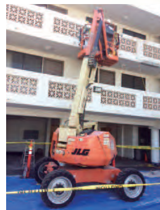
The BDK Hawaii building is under repair
