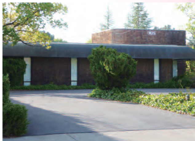
Front view of new office building in Moraga
